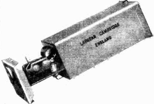
Makes an outstanding improvement against interference from transmitters on frequencies lower than the TV channels. One required for co-ax aerial feeders, two for balanced twin-lead. Price 10/6, plus 9d. P./P. only, direct from.
