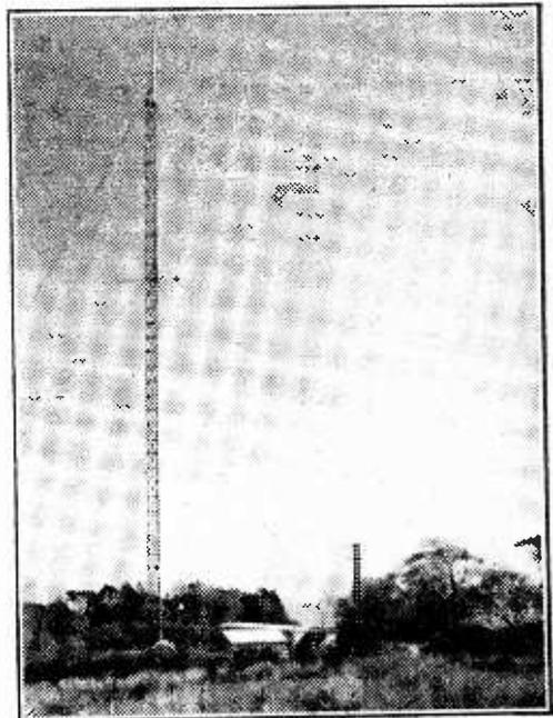
The 235ft. mast with 23½ft. single-stack super turnstile aerial, horizontal polarisation, which Marconi's Wireless Telegraph Co. Ltd. erected at Glencairn Road, Belfast, in time for the Coronation.
