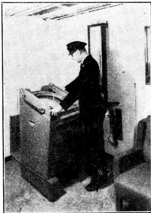
The new Orient liner, "Orsova," is the first ship to have the new Marconi Marine 15in. "Radiolocator" radar. One of the "Orsova's" navigating officers is seen watching the screen of the new radar in the liner's chartroom.
