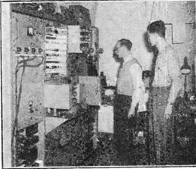
The flying spot film scanner used to show "still" images at the demonstration.
