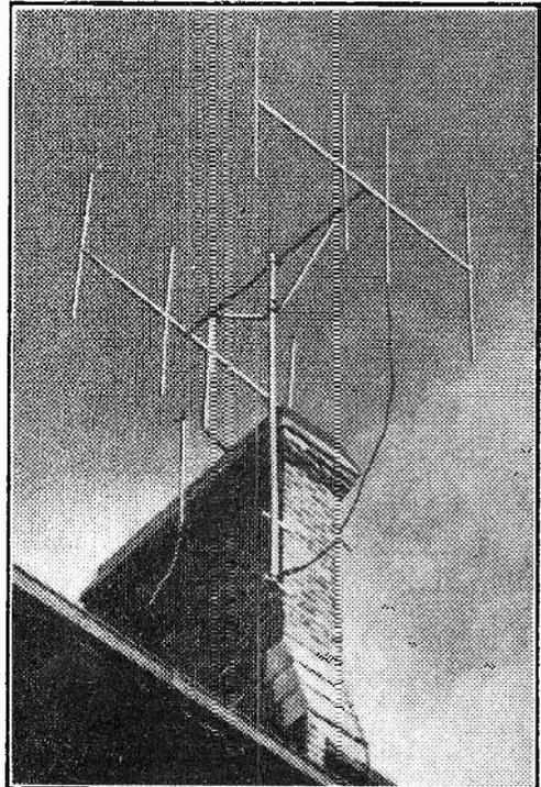
Fig. 59.—This type of double four-element aerial system is often essential for good pictures in fringe areas.
