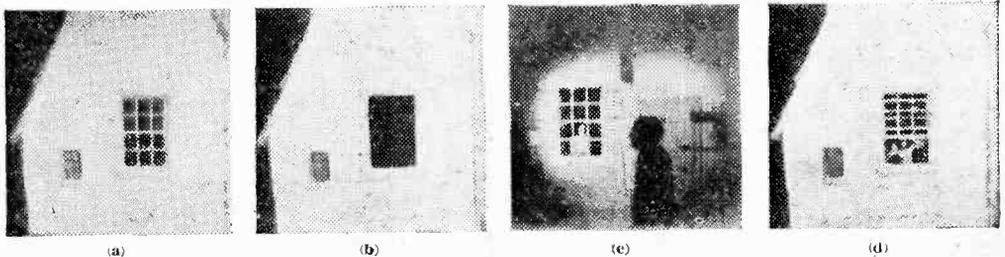
Fig. 3.—How the producer sees an Inlay effect on monitor screens.
