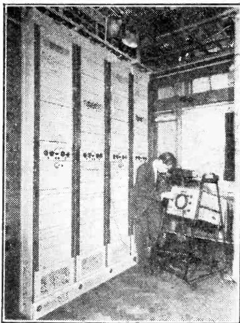
An operator uses an oscilloscope to check a panel on a two-channel transmit terminal at Telephone House, Birmingham. (See "Two ITA Links.")
