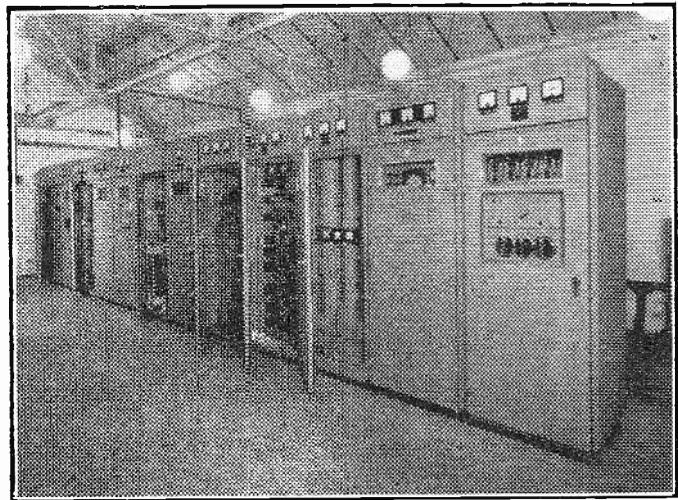
Marconi Vision and Sound Transmitters as used at ITA London and Winter Hill. The  $7\frac{1}{2}$  kW vision transmitter occupies the first seven panels from the right; the  $2\frac{1}{2}$  kW sound transmitter the remainder.
