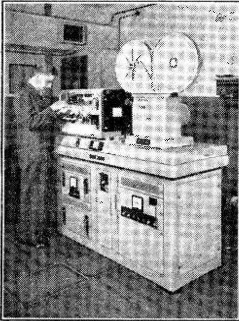
A general view of the new Marconi Telerecording Equipment with an engineer examining the underside of one of the sub-chassis from which the covers have been removed. A feature of the equipment is the way in which the sub-chassis are hinged, so that access to units is facilitated and servicing very much simplified.
