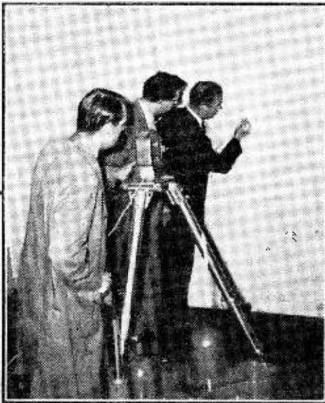
Such is the accuracy required in the floor level of a modern television studio that tests, such as this picture shows, must be made before the floor can be declared "ready for action." A slide projector, mounted on a mobile pedestal, casts a beam of light on to a line drawn round the walls of the studio at a standard height from the ground, and the light should remain on this line as the pedestal is tracked round the studio.
