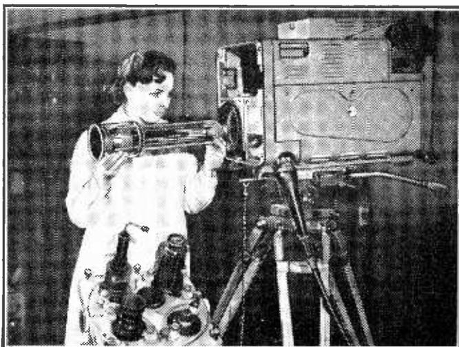
A 4½in. Image Orthicon tube being fitted into a Marconi Mk. III camera. See "Canada Buys British" above.
