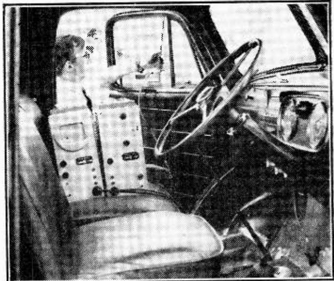
Television is being employed by Vauxhall Motors to test car behaviour under varying conditions. (See page 493.)
