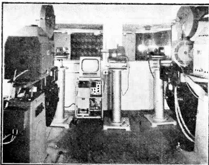
The projection room of L.P.E. Television Ltd., with two Marconi BD871 television cameras mounted on pedestals for telecine work. (See "Closed Circuit Television".)
