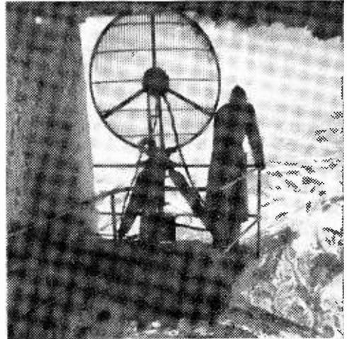
This view shows a portable "mirror" directed at the valley below, where a mobile television unit is transmitting.
