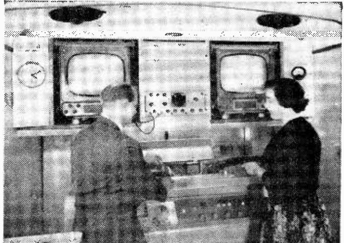
Mr. Walter Kemp, Technical Controller of TWW, loads the two-inch wide magnetic tape on to the video and audio record heads for recording in the new specially-designed mobile Ampex videotape recording unit. This unit, which has just been delivered to TWW, will be used for recording studio programmes and outdoor events in Wales and the West Country. This picture gives a close-up of the Ampex console with the record and preview picture monitors on each side of the waveform monitor.
