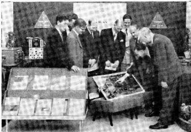
A group of interested visitors examine an "S" band power distribution board engineered in high Q triplate strip transmission line and exhibited at the 1959 Farnborough Air Show. The double-sided board, designed by Cossor Radar and Electronics, Ltd., was printed and etched to extremely fine limits by Printed Circuits, Ltd., of Borehamwood. It houses 32 "S" band components consisting of branch arm and proximity couplers, cross-over network matched loads, and variable attenuators.
