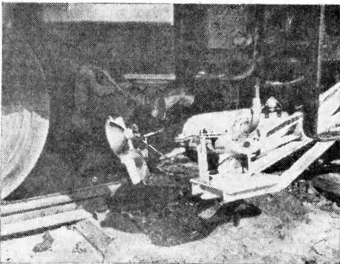
Following abnormal wear on sharp curves on some railway tracks, Rhodesian Railways mounted a closed-circuit TV camera on a locomotive so that the action of the wheels could be observed (see "TV for Rhodesian Railways").
