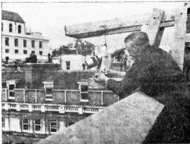
Taylor Woodrow Ltd. have installed Marconi closed circuit television on the site of the new building they are erecting at the junction of Gracechurch Street and Fenchurch Street. The installation enables the public to watch building operations in progress on a 21in. monitor fitted in a public observation platform. This illustration shows a Marconi engineer fitting the closed circuit television camera on the roof of a building adjoining the site.
