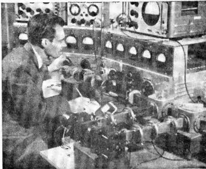
In the Radio Communications Group (G.E.C. Research Laboratories), an engineer assesses the performance of a travelling wave amplifier, type TWCS. This device has been specially developed for a wideband microwave radio system—the first planned to operate in this country in the 6,000 Mc/s band. The system has already been chosen for the new British television link between Carlisle and Kirk o'Shotts.
