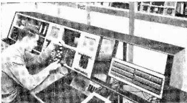
*A telecommunications worker assembling one of the nine broadcasting control desks. From these desks is controlled the quality of radio and television transmissions. All desks have equipment prepared for the transmission of stereophonic sound and colour television.*
