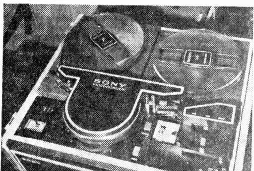
Top deck view of the Sony CV2100 recorder. The edit and dub buttons are next to the record button.
