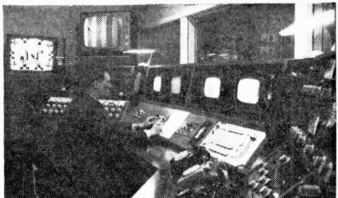
*Telecine Control Room: In the foreground the audio test selector, tone generator and channel control panels. In front of the controller are the four video monitors, camera control units and mixing panels. Beyond the controller are the intercom waveform monitor and relay selector panels. Above these can be seen the R.G.B and black-and-white terminal monitors.*
