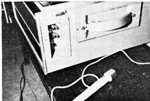
The standby switch with other selectors is sited in a recessed panel at the right-hand side of the recorder, the slave machine, giving effective duplication. And a camera signal can be recorded simultaneously on the two machines.
