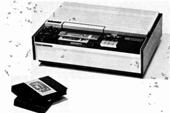
*The Sony U-matic colour videocassette machine. There are two versions: the VO1601D has both recording and playback facilities while the VP1001D is for playback only. An optional r.f. unit is available. A rotary two-head helical-scan system is used and the luminance signal is frequency modulated.*
