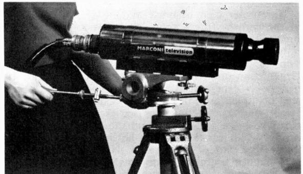
Fig. 1: A typical separate-head camera, the Marconi CCTV camera type V321.
