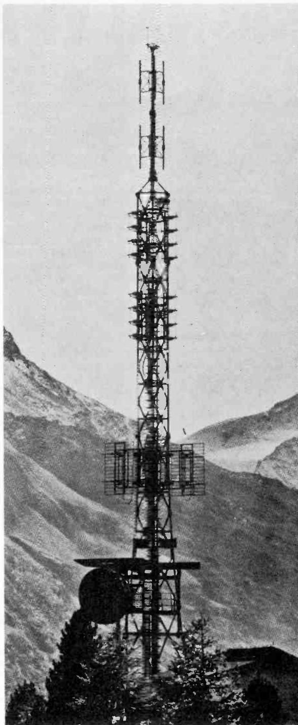
*The Monte Celerina, Switzerland transmitter, at 2100 meters a.s.l. Ch. E7 3kW Italian; ch. E9 6kW German. Photograph courtesy Radic Electronics, Holland.*
