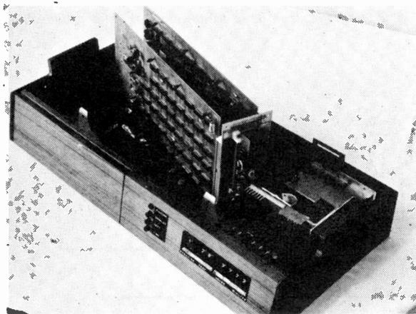
Internal views of GEC's experimental Ceefax/Oracle decoder.
