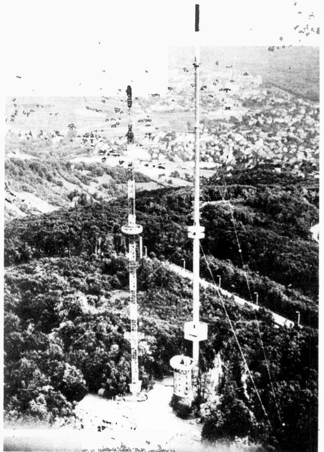
The Vienna (Austria) transmitter mast has recently been replaced by ORF to improve the coverage. The new (right) and old (left) masts at Kahlenberg are shown here. The v.h.f. aerial structure was lifted one metre to 123m; the u.h.f. aerial structure was raised from 65m to 152m. The u.h.f. panels can just be seen below the circular platform of the old lattice structure.
