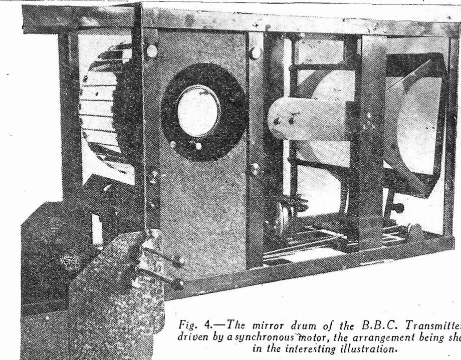
Fig. 4.—The mirror drum of the B.B.C. Transmitter is driven by a synchronous motor, the arrangement being shown in the interesting illustration.
