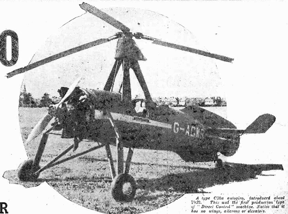
A type C30a autogiro, introduced about 1932. This was the first production type of "Direct Control" machine. Notice that it has no wings, ailerons or elevators.
