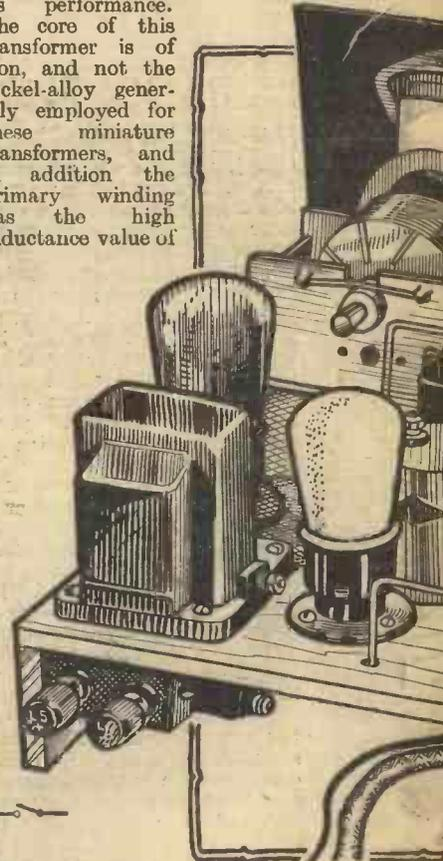
The battery-operated Fury Four can be converted to A.C. operation by the addition of the components illustrated.
