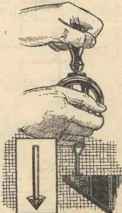
Fig. 2.—Countersinking an ebonite panel.
