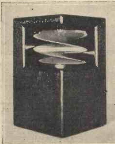
Fig. 2.—Showing very clearly how the mirror screw is built up like a spiral staircase.
