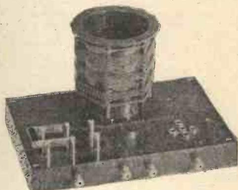
The Eelex short-wave converter chassis.
