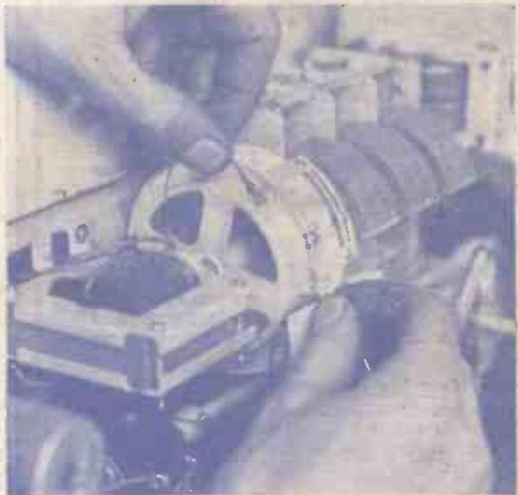
Another splendid illustration showing the fitting of a New Cord to the Drum of the Marconiophone 42 Receiver.
