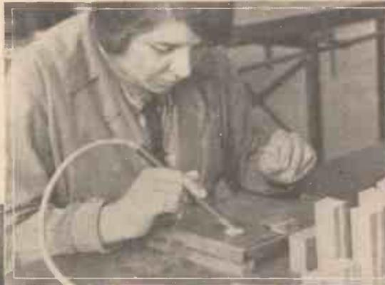
Fig. 1 (above).—Testing mica for insulation.
