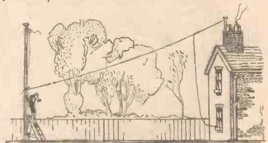
Fig. 1.—Fixing a fallen aerial at "half-mast" as a temporary measure.
