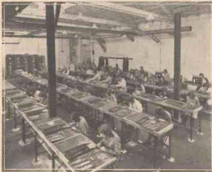
Fig. 4.—Assembling fixed condensers in the factory.
