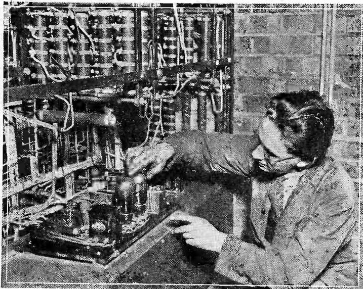
A new system of gearless drive has been introduced to England for the first time in a London building, where sixteen new lifts have just been installed. The interesting feature of this system is that two thermionic valves, such as are used in ordinary wireless sets, smoothly control the stopping and slowing of the lifts. The illustration shows an engineer replacing one of the thermionic valves.
