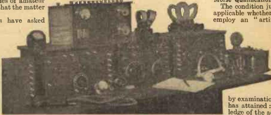
The above photograph shows a typical amateur transmitting station; the photograph was taken a few years ago, and this accounts for the use of plug-in coils.
