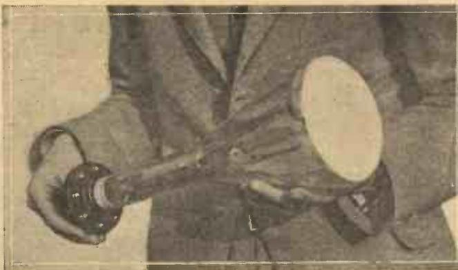
Fig. 1.—A standard form of cathode-ray tube, showing clearly the front fluorescent screen where the television image is built up.
