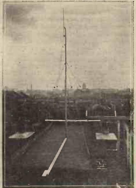
Fig. 3.—Showing the high situation of the first dipole aerial erected for an ultra-short-wave demonstration in 1932.
