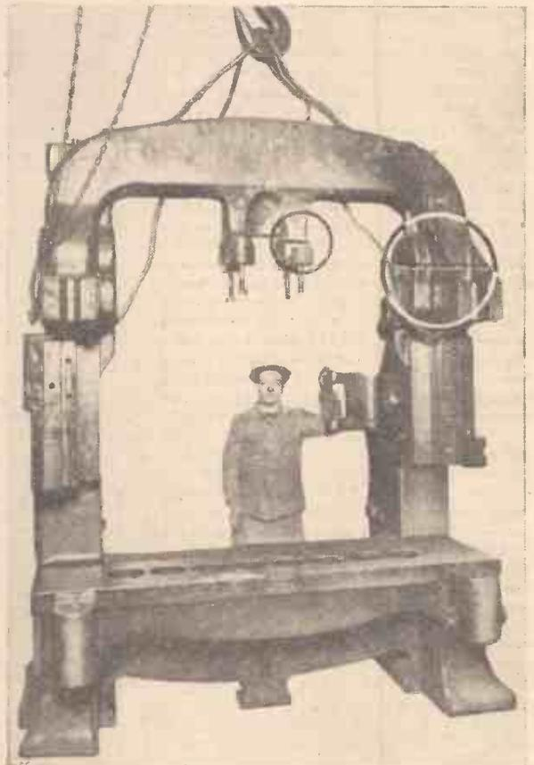
This illustration shows the cracks in a powerful press which were repaired by the low-temperature welding process described in this article.
