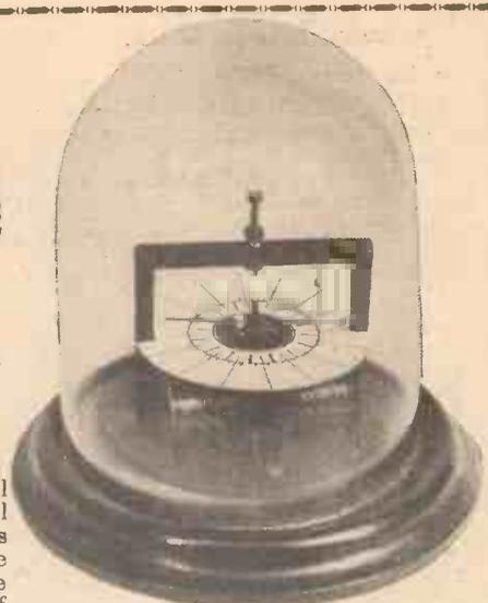
The finished galvanometer.
