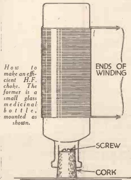
How to make an efficient H.F. choke. The former is a small glass medicinal bottle, mounted as shown.
