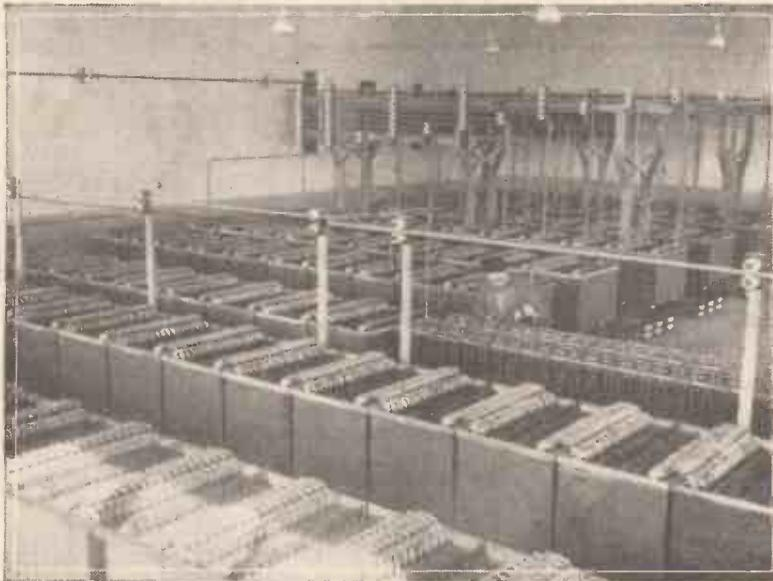
At the new radio station at Severac a large bank of accumulators is maintained, and a section of these may be seen in this picture.
