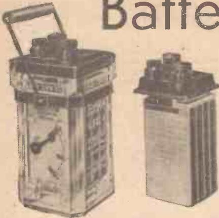
The Exide "Hycap" accumulator ready for use and with the plates withdrawn.
