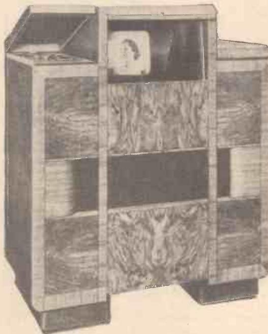
In this Marconiphone television receiver a vertical tube is used, and the image on the end of the tube is viewed in a mirror.
