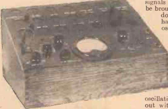
For the service-man, an all-valve tester of this type will be found essential in tracing faults and saving time.
