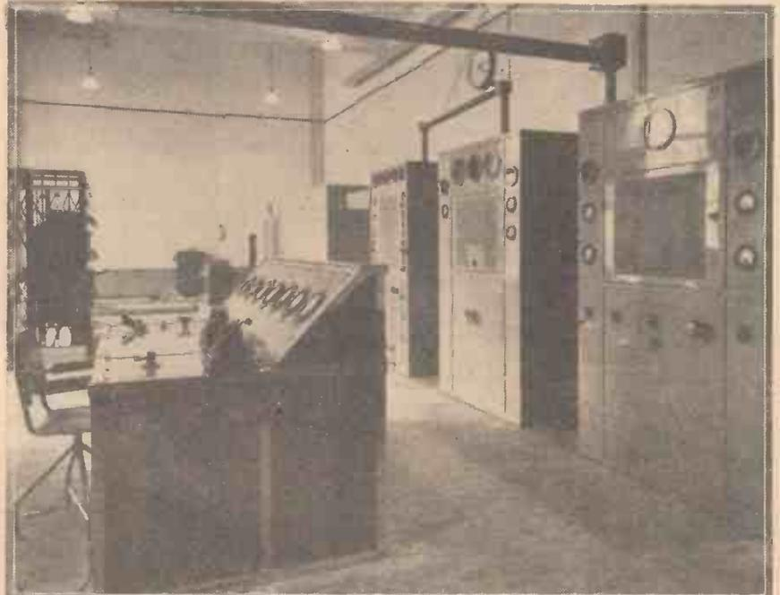
Alexandra Palace Television Station B.B.C. sound transmitter. Control table—left foreground. Drive unit and low power H.F. stage—centre background. Final power amplifier—centre right. Modulator unit—right. Power switchboard—left background.
