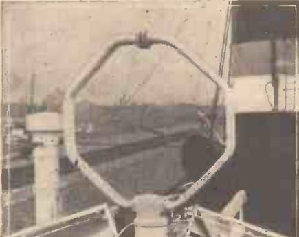
The G.R.C. Auto-alarm for the reception of distress signals is an entirely self-contained equipment. It also embodies means for automatic transmission which will continue as long as power is available. A high degree of reliability is obtained owing to the absence of any continuously rotating mechanism or motor-driven parts, movements only occurring when signals are being received.
