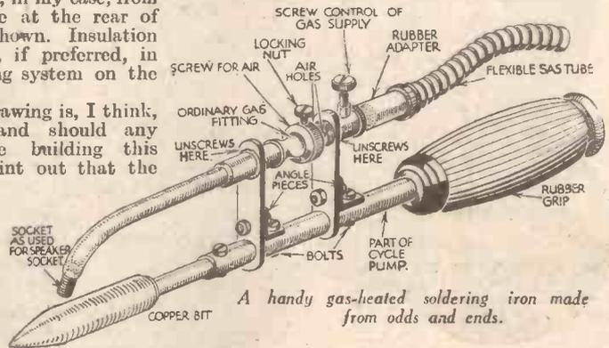
A handy gas-heated soldering iron made from odds and ends.
