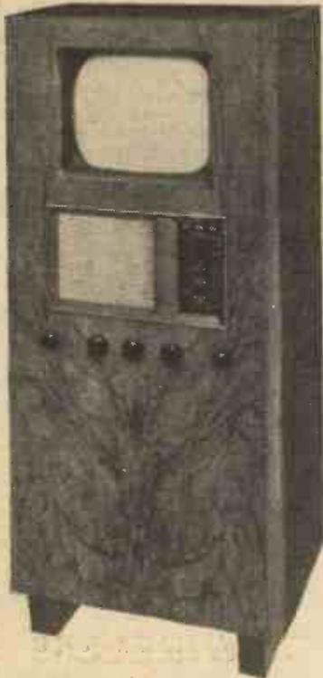
One of the new Baird television receivers which combines an all-wave radio receiver.
