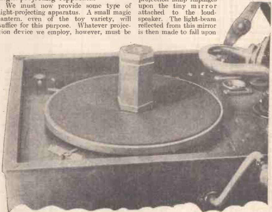
*The home-made six-sided mirror-drum of the oscillograph mounted on the spindle of a gramophone turntable. The mirrors are secured in position on the supporting block by means of rubber bands.*
