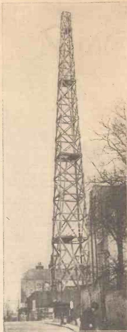
A new television mast 150 ft. in height is now being erected for the outside broadcasts of television. The existing aerial at Alexandra Palace interferes with other programmes. This one, on the top of Highgate Hill, will be well away from any interference.
