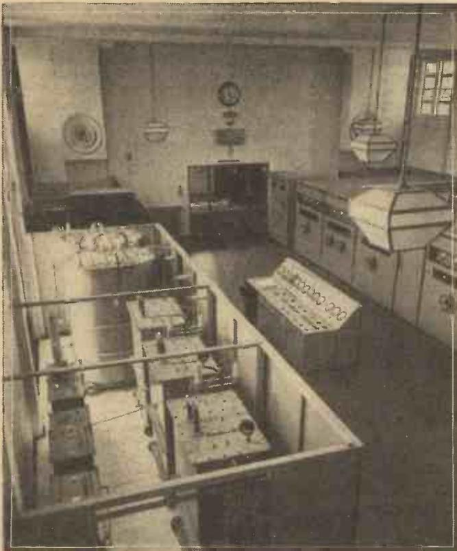
Above is the Transmitter Hall of Start Point Transmitting Station, seen from the gallery. The transmitter centre and control desk is on the right, and on the left the modulation transformer and plate feed reactors. The picture on the right shows the station buildings and masts.
