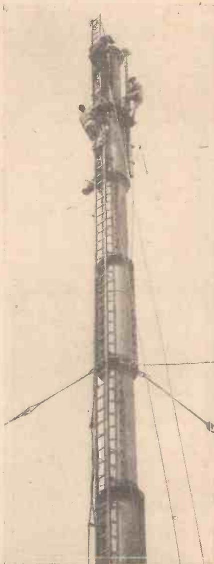
The steeplejacks are now busy at work demolishing the 240 ft. steel aerial mast over the Marconi experimental station at Chelmsford, which is being dismantled. Our illustration shows a precarious perch for the workmen at work on the top of the aerial mast.
