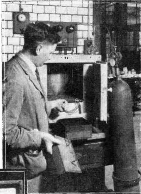
Fig. 2.—The perishability of rubber insulation is quickly gauged by accelerated life test to which it is subjected in the chamber of this humidity cabinet.
