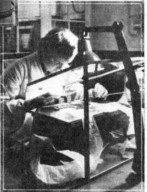
Fig. 4.—Even the breath of the operator is shielded from the work in this air-conditioned assembly room.
