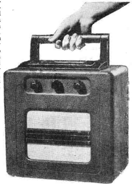
*The Ekco "Pick-me-up" portable—an 8-stage superhet. It measures 11½in. by 11½in. by 7½in.*
