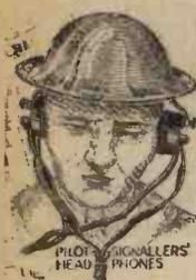
**SERVICE SIGNALERS' DOUBLE HEADPHONES.** With flat leather headbands for steel helmet wear, 120 ohms, by S.T. Co., 3/8, 4ft. cords. Single 60 ohm. phones with cord D.L.I. 1/6. **FIELD Telephone Exchanges.** 5-line and 20-line portable. Twin and single cable. **HEADPHONE CORDS.** Service 8ft. fitted 2-pin. plugs and 2-hole socket, 2/- **Radio Phone Cords.** 2/6.
