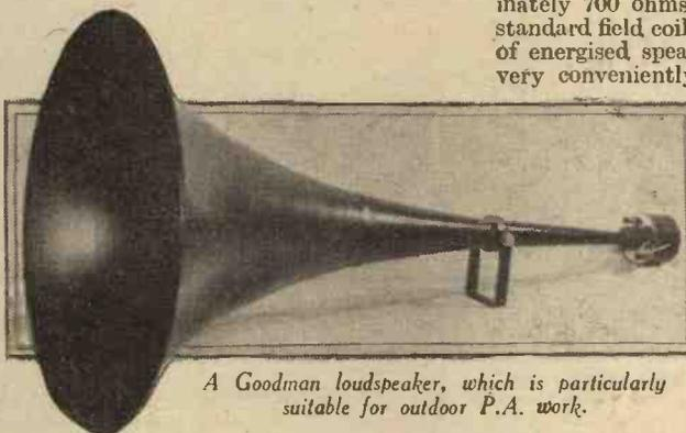
A Goodman loudspeaker, which is particularly suitable for outdoor P.A. work.
