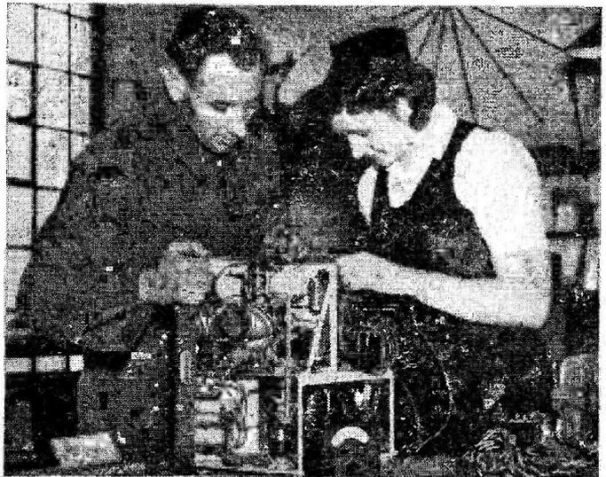
An A.T.S. girl working with a soldier on overhauling and repairing transmitting and receiving sets.
