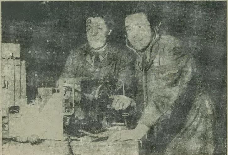
A.T.S. twin sisters M. and V. Hills, testing portable wireless sets used by the Army.
