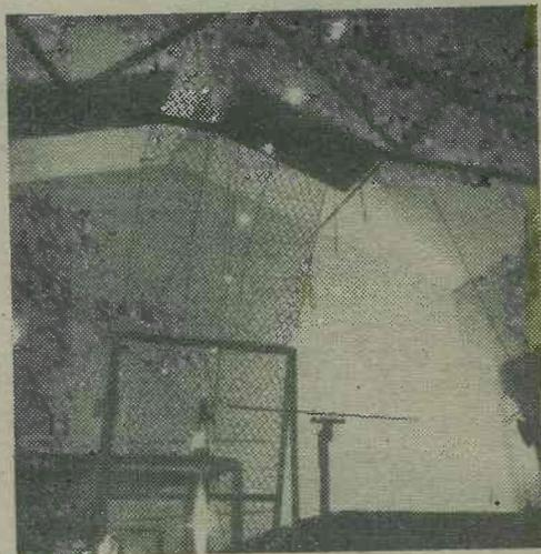
Fig. 3.—Polar diagram of dipole aerial. The brightness of the various lights indicates comparative strength of radiation in different directions.
